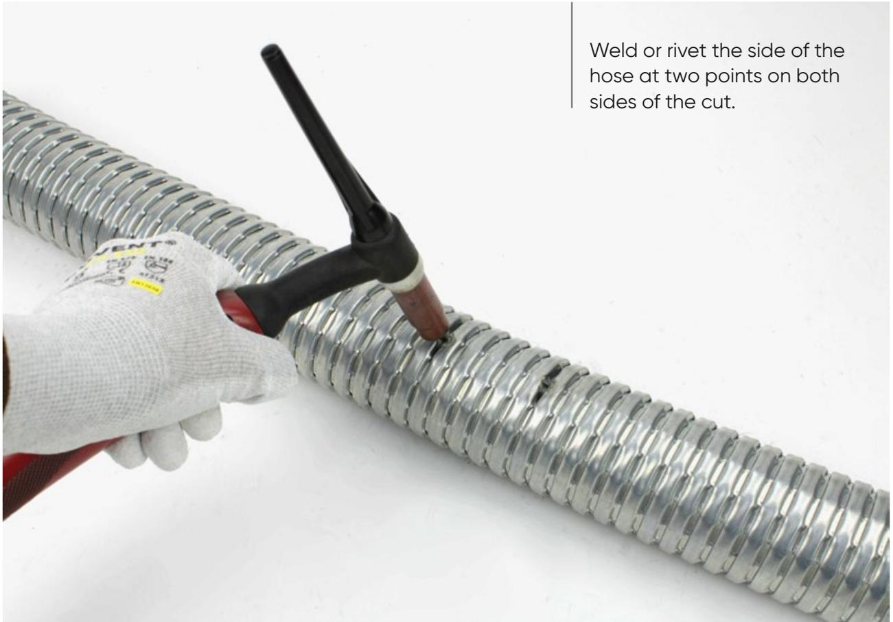
Weld or rivet the side of the hose at two points on both sides of the cut.
